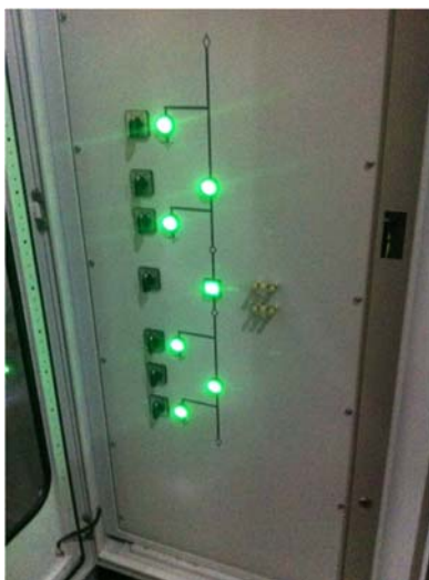
Figure 2-44 Schematic diagram of main connection simulation
